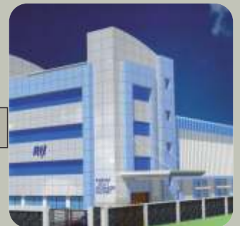
Radiant Heat Exchange Pvt. Ltd
